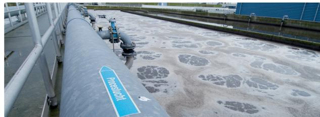
Many WWT plants use aerobic biological processes to digest waste by-products. Typically, the major energy consumers in these plants are the aeration blowers. To permit energy optimization and substantially reduce energy bills in these continuously operating plants, Atlas Copco's innovative ZS blowers incorporate the latest technologies in the most efficient design.
